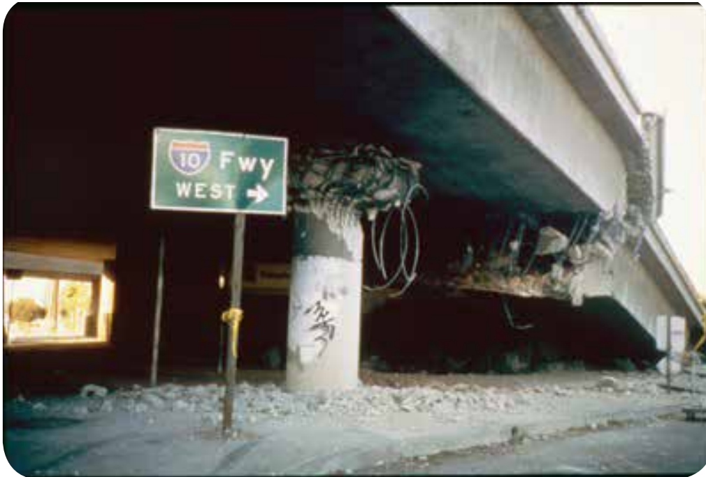
Northridge Earthquake: Interstate 10 bridge collapse at La Cienega Blvd (photo from Stewart et al., 1994; EERC Report 94/08) Northridge20 Symposium at UCLA on Jan. 17, 2014.
