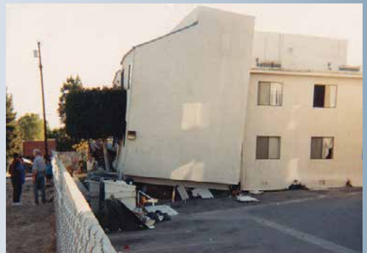
An apartment building in Reseda, CA in January of 1994 after the Northridge Earthquake. Photo: Eric Gelinias via Flickr Creative Commons
