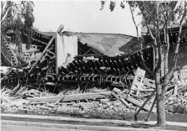
Long Beach, California, Earthquake March 10, 1933. View showing damage to Jefferson Junior High School. Photo from Capt. T.J. Maher, Coast & Geodetic Survey.
