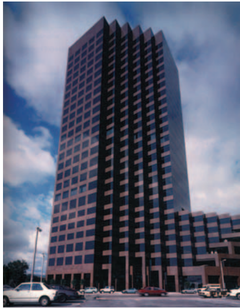
Figure 2. Twenty-seven-storey building near Wilshire Blvd and Barrington Ave. (view 2)
