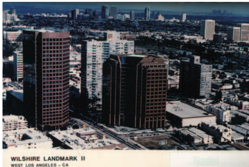
Figure 1. Twenty-seven-storey building near Wilshire Blvd and Barrington Ave. (view 1)
